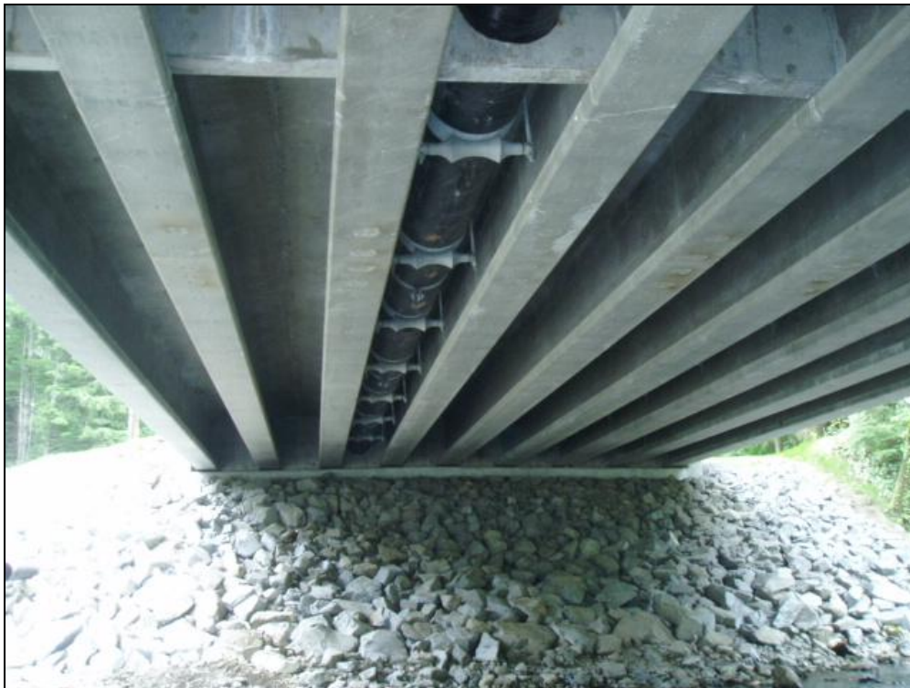
Figure 4 New High Density Polyethylene Piping on Indian River Bridge
