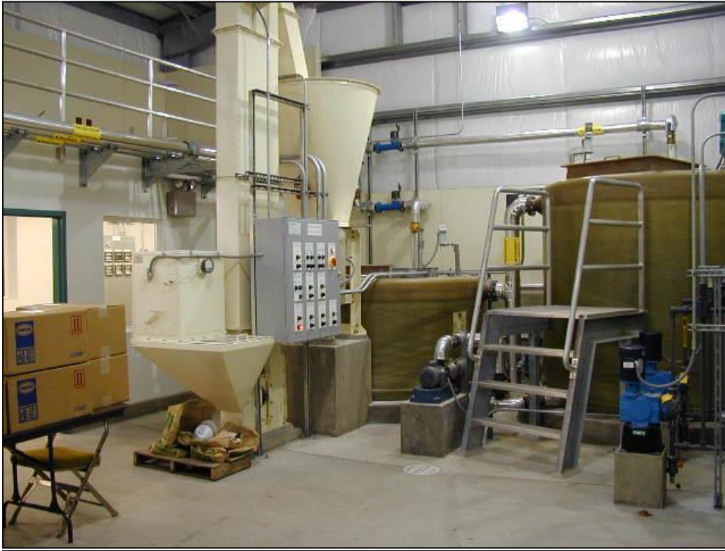
Figure 5 Corrosion Control Facility on Jarvis Street
