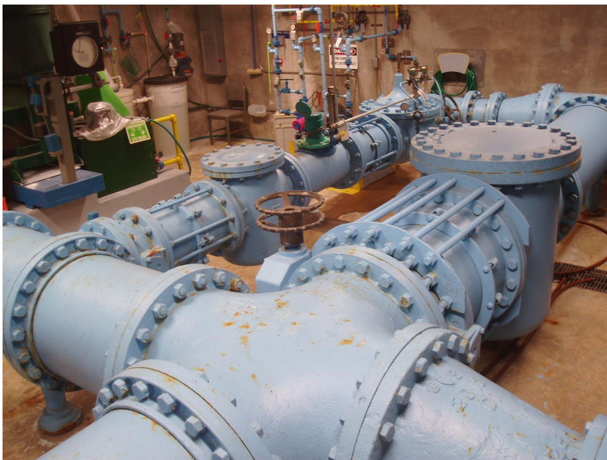
Figure 3 Flow Control Valves at Blue Lake Water Treatment Plant
