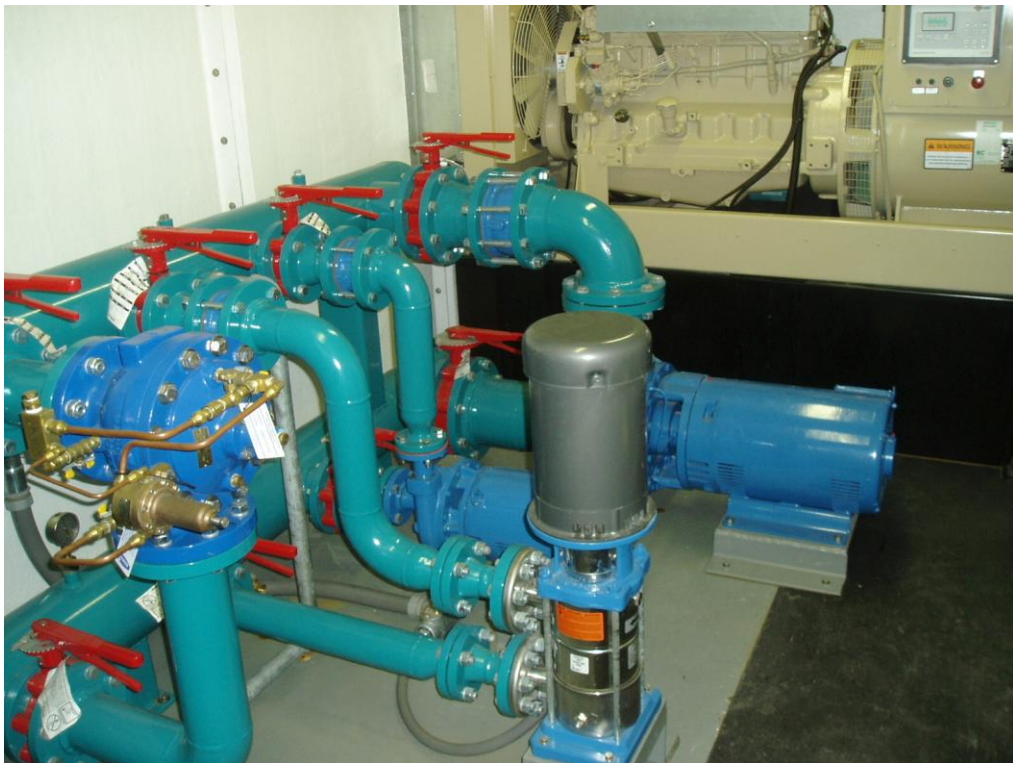
Figure 9 Hillside Water Booster Pump Station
