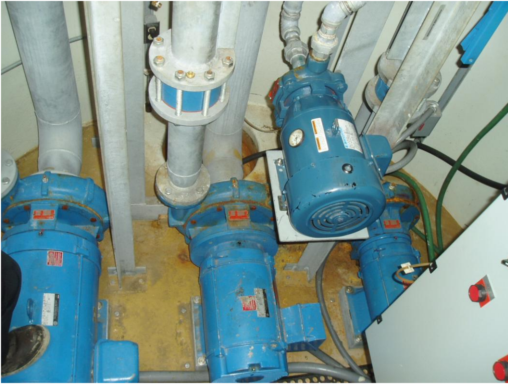
Figure 8 Wortman Loop Water Booster Pump Station
