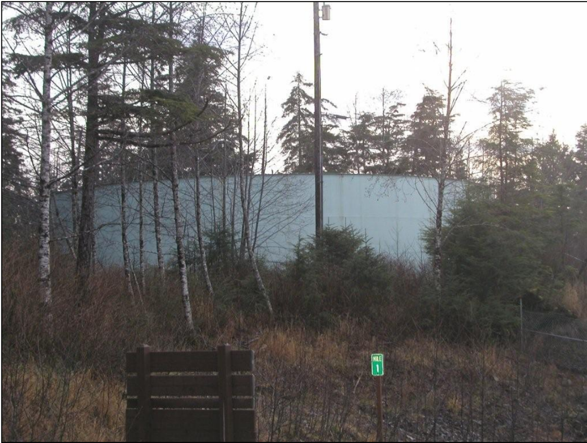
Figure 6 Harbor Mountain Water Tank (0.75 MG)
